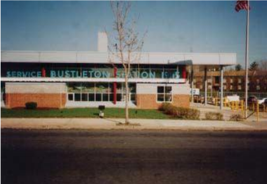
Exhibit 2 Building - West Elevation – Close Range
