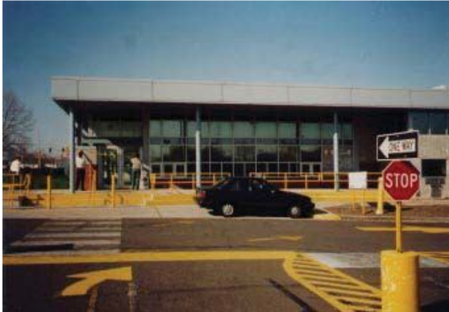
Exhibit 3 Building - South Elevation – Close Range
