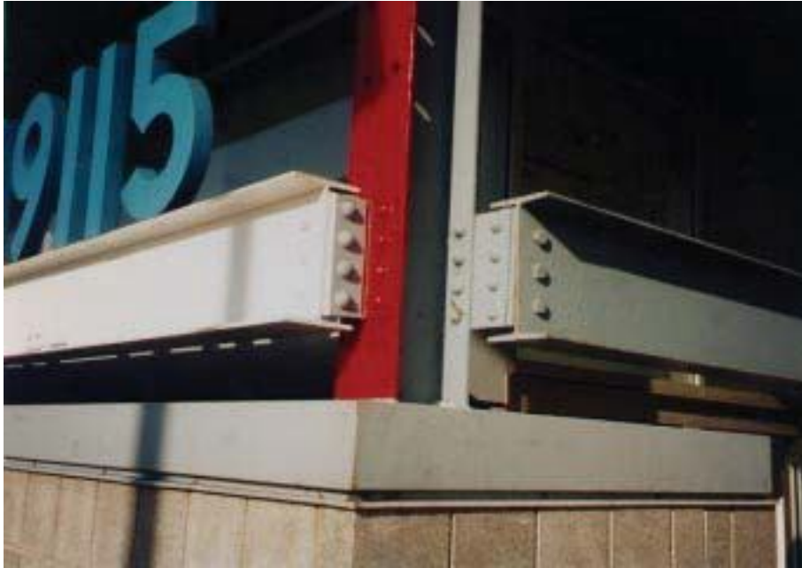
Exhibit 5 Building Construction - Detail Shot
