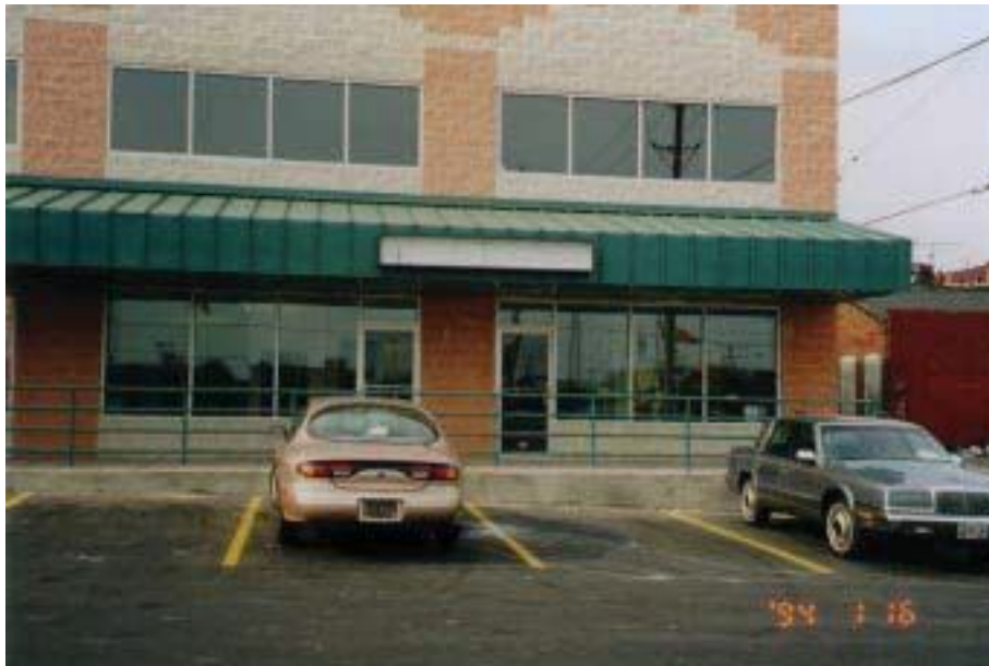
Exhibit 8 Building – South Elevation – Close Range
