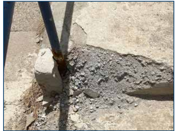
Crumbling concrete
