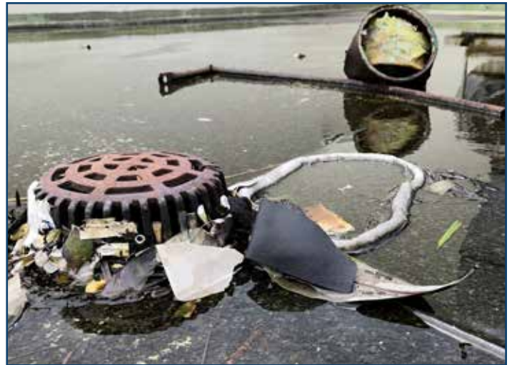
Sieves over drains collect debris and should be cleaned often.
